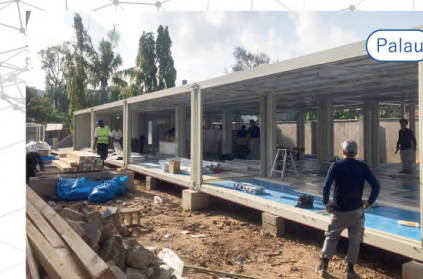
Remote ICU prefabricated ward, etc. installation
