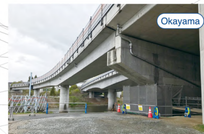
Sanyo Expressway seismic retrofit
