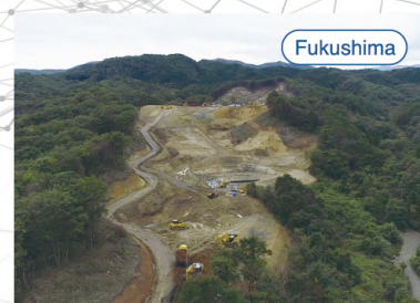
Koriyama site development 2.4 million m 2
