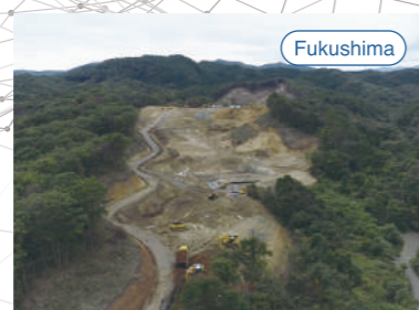
Koriyama site development 2.4 million m 2
