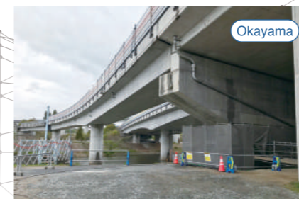
Sanyo Expressway seismic retrofit
