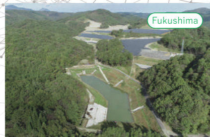
Construction of a 20 MG solar power generation plant in Shirakawa, Fukushima
