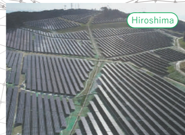
Construction of the Hatsukaichi City 44 MG mega solar plant
