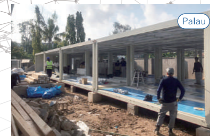
Remote ICU prefabricated ward, etc. installation
