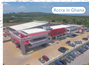
TOYOTA GHANA WORKSHOP AND UG ENGINEERING TRAINING CENTRE
