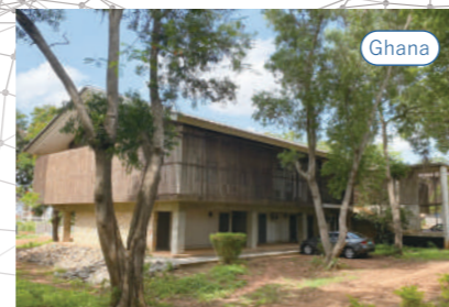
Air conditioning equipment repair work for Noguchi Memorial Institute for Medical Research
